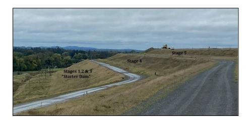
Figure 6.2: Embankments side profile
