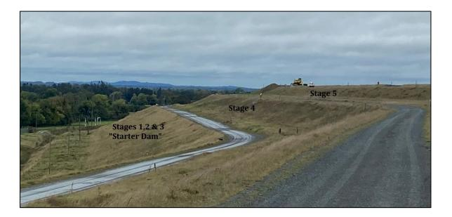
Figure 6.13: Stages 1 to 5 Embankments - side profile
